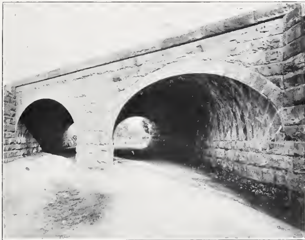
MASONRY-SKEW ARCHES Lake Shore Railway Bridge over Lake Avenue
